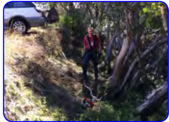
Blair Hume (access track construction)
