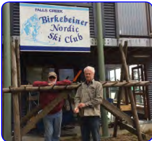
Brian Keeble & Doug Hamilton (Sign erection & ski rack repairs)
